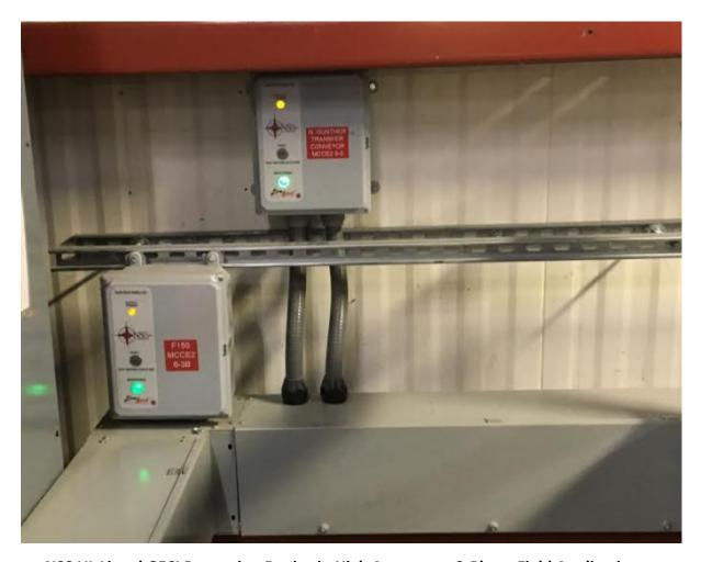
NSS UL Listed GFCI Protection Device in High Amperage, 3-Phase Field Application
